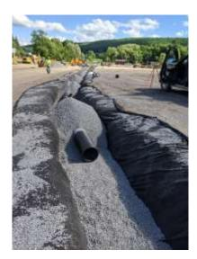
(LD) This is the perimeter drain. It is perforated pipe. As you know you had a lot of storm water and ground water problems on this site, so the whole field was raised, I would say an average of 2-2-1/2'. So about 10,000 cubic yards of structural fill was brought on the site.
