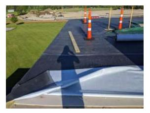
any of that roofing material, new insulation and new layer of rubber EPDM roofing was installed.
