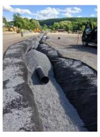
(LD) This is the perimeter drain. It is perforated pipe. As you know you had a lot of storm water and ground water problems on this site, so the whole field was raised, I would say an average of 2-2-1/2'. So about 10,000 cubic yards of structural fill was brought on the site.
