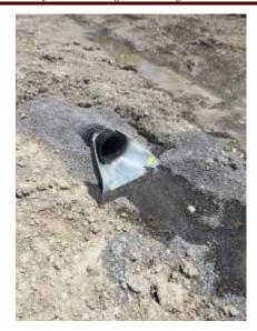
This is today – in all this heat – and I don't know if you can see it – but there's probably an inch of flow in that discharge pipe into the swale that leads off site. So even in the driest of times you have a pretty steady flow of ground water and it is cold. It is cold to the touch. It is interesting but it is continuous and even in almost drought-like conditions.
