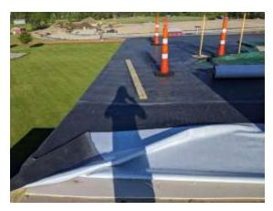
roofing material, new insulation and new layer of rubber EPDM roofing was installed.
