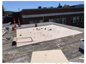
So what you see here is the top layer of roofing as well as the insulation down to the roof deck was removed. It was saturated beyond really repair. So CJ Marley removed 2 problem areas approximately 15' x 20' give or take, which were known to be causing leaking in the gymnasium. And then installed poly.....insulation, as well as blocking around the perimeter of the roofs obviously and then a new rubber roofing system
