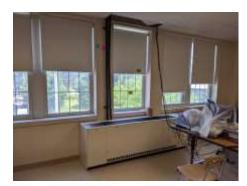
So, this is just a photo of one of the typical unit ventilators as it is installed right now. The piping you see against the wall there is refrigerant piping that goes up through the ceiling, out into the corridor, then penetrates up through the roof to the condensing units up there. Currently we are just waiting on control wiring to be installed to these and then pipe covers on that insulated pipe and then installation of these will be effectively complete.
