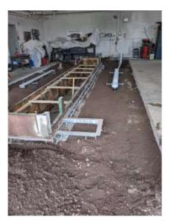
Current the bus lift installation is complete and it is being used every day by the mechanic here. We were fortunate enough to get an early start on that work back in early May. So installation of the Bus Lift involved the removal of the existing lift as well as demolition of the existing slab, new
